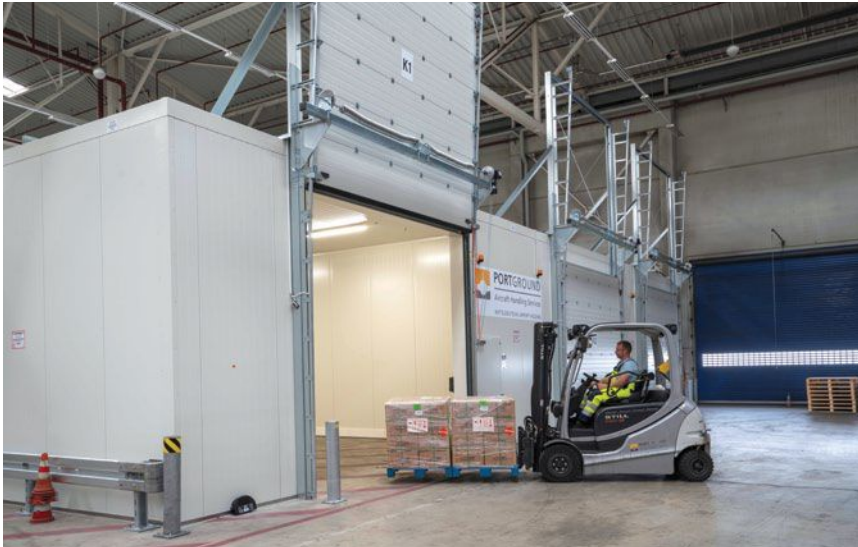
Refrigerated warehouse for air freight at Leipzig Halle Airport
